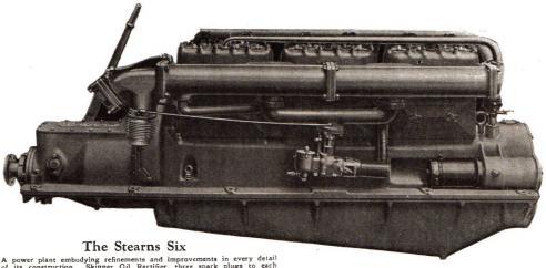
A power plant embodying refinements and improvements in every detail of its construction. Skinner Oil Rectifier, three spark plugs to each cylinder, two independent ignition systems and high pressure lubrication are only a few of the major improvements the Stearns gives you.
